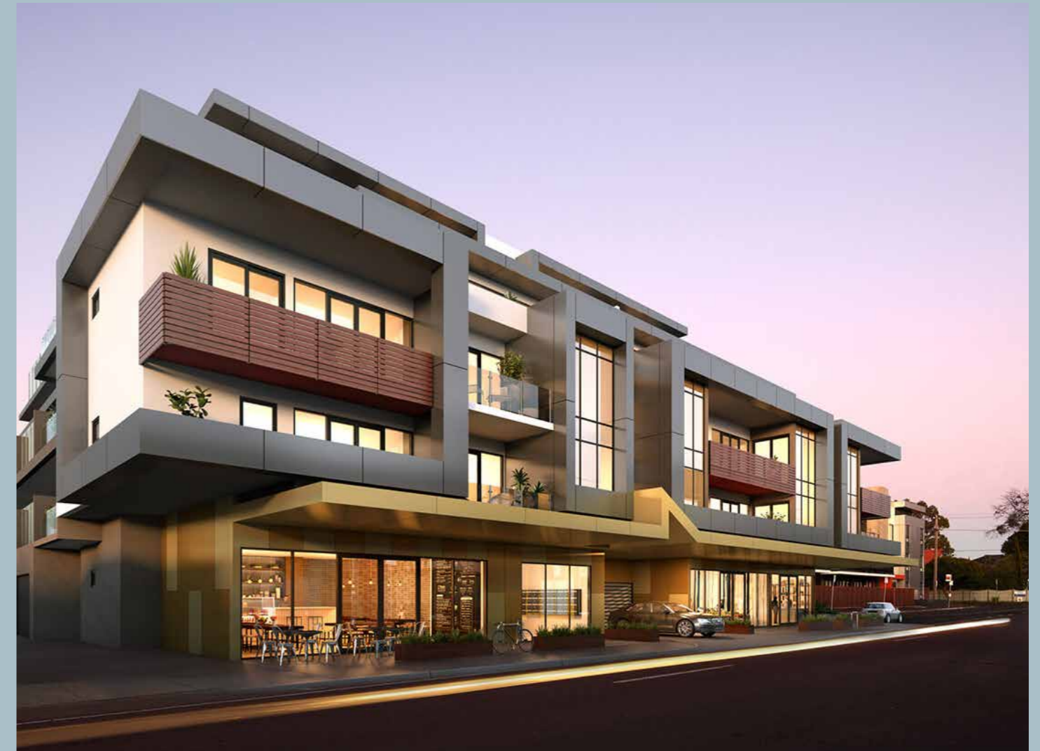
Portal Apartments, Carnegie, Grand Properties Consortium
